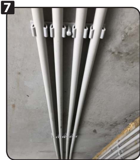
The tubes are positioned !
